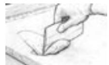
When using the wet method, it may be advantageous to cut the fabric once wetted out. This will ensure accurate placement of the fabrics and stability of the cloth from the roll. Use an adapted clothes rail, taught, rope or a broom handle to allow free dispensing of the cloth from the roll. Clean scissors etc, with 850 cleaning solvent.
